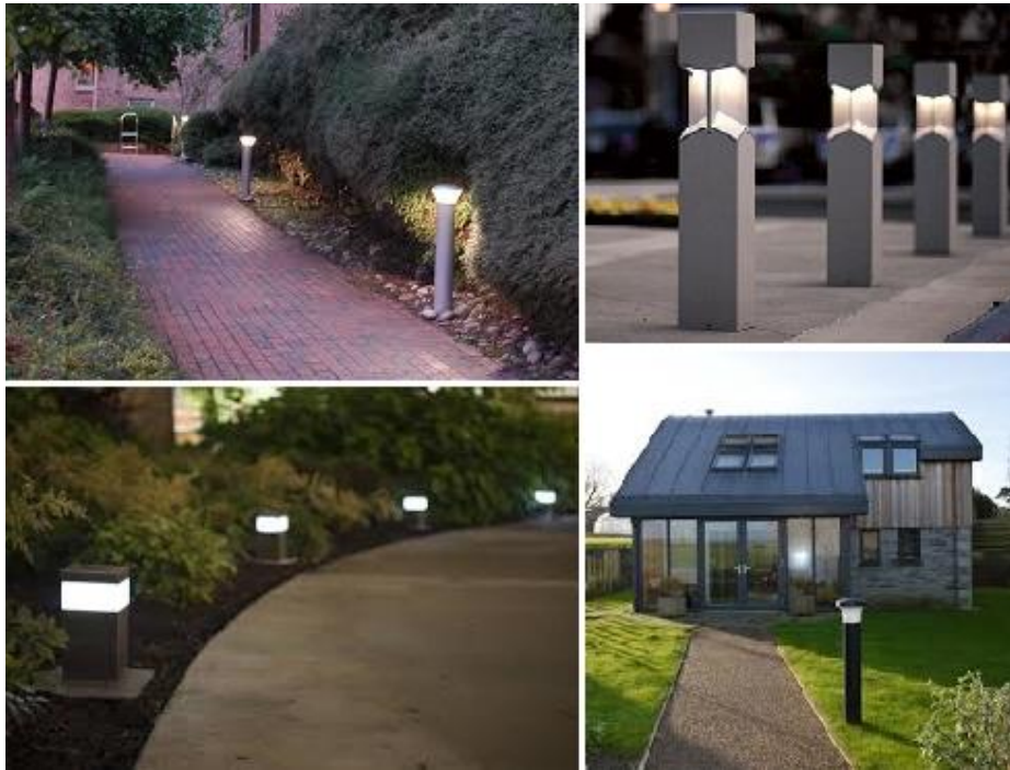
Figure 5-20: Examples of Pedestrian Bollard Lamps
